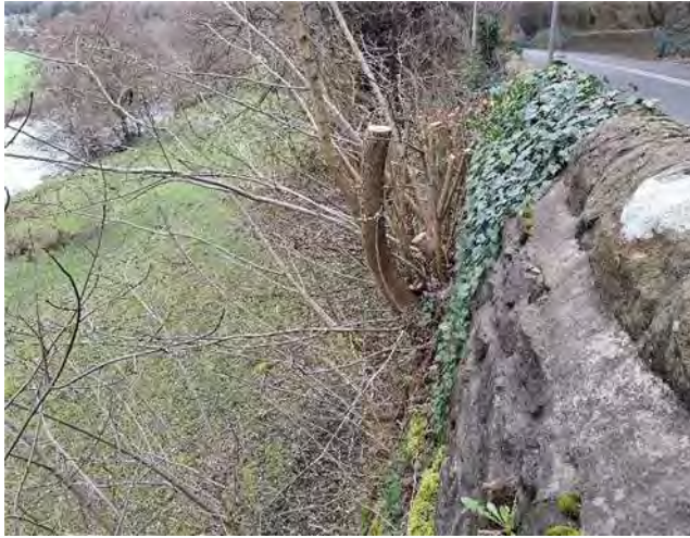
Retaining Wall (Primary)
