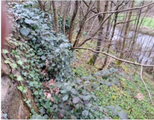
Retaining Wall (Primary)
