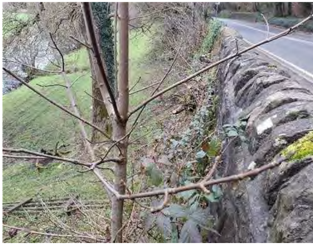
Retaining Wall (Primary)
