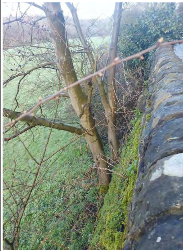
Retaining Wall (Primary)
