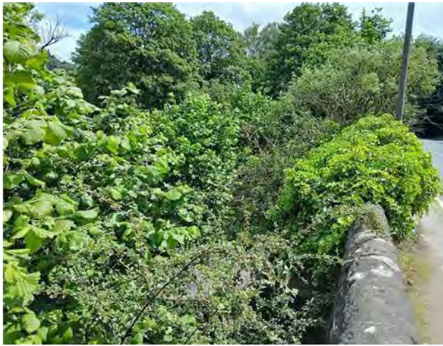
Retaining Wall (Primary)
