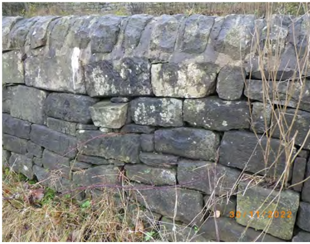
Retaining Wall (Primary)
