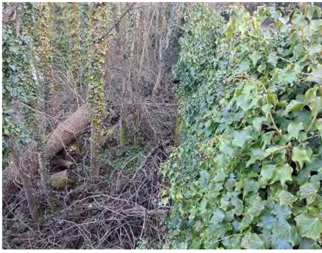
Retaining Wall (Primary)
