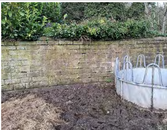
Retaining Wall (Primary)
