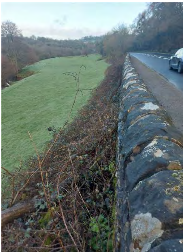
Retaining Wall (Primary)
