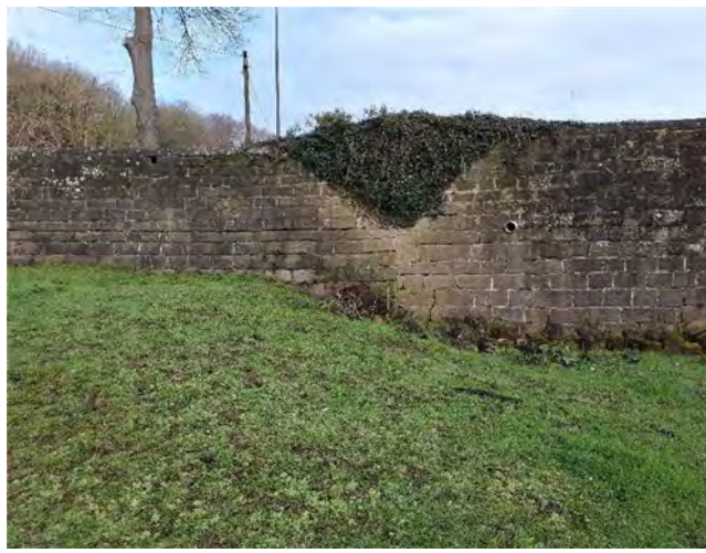
Retaining Wall (Primary)
