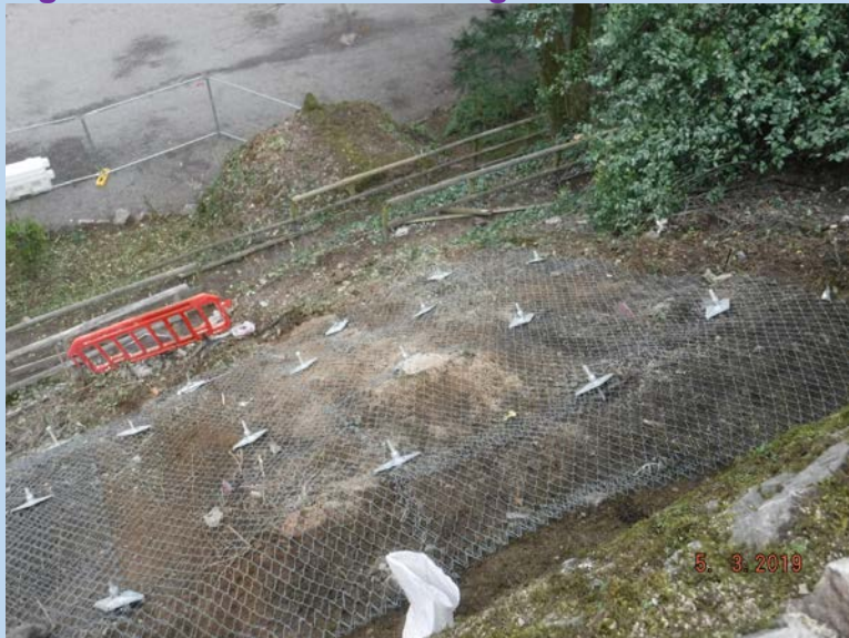
Figure 4 – Soil Nails to Strengthen Embankment
