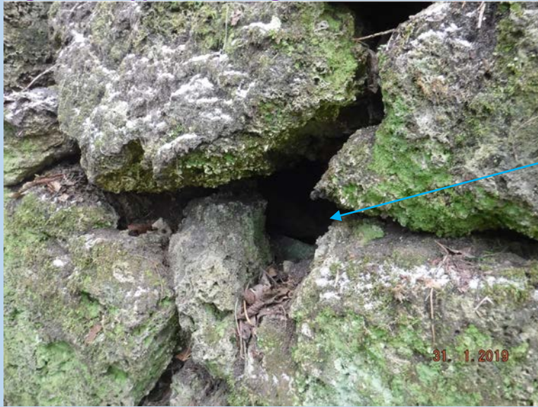
Figure 3 – Typical Voiding of Wall and Foundations
