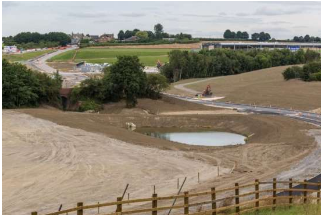
Earthworks, road construction and development building contractors all working together.
