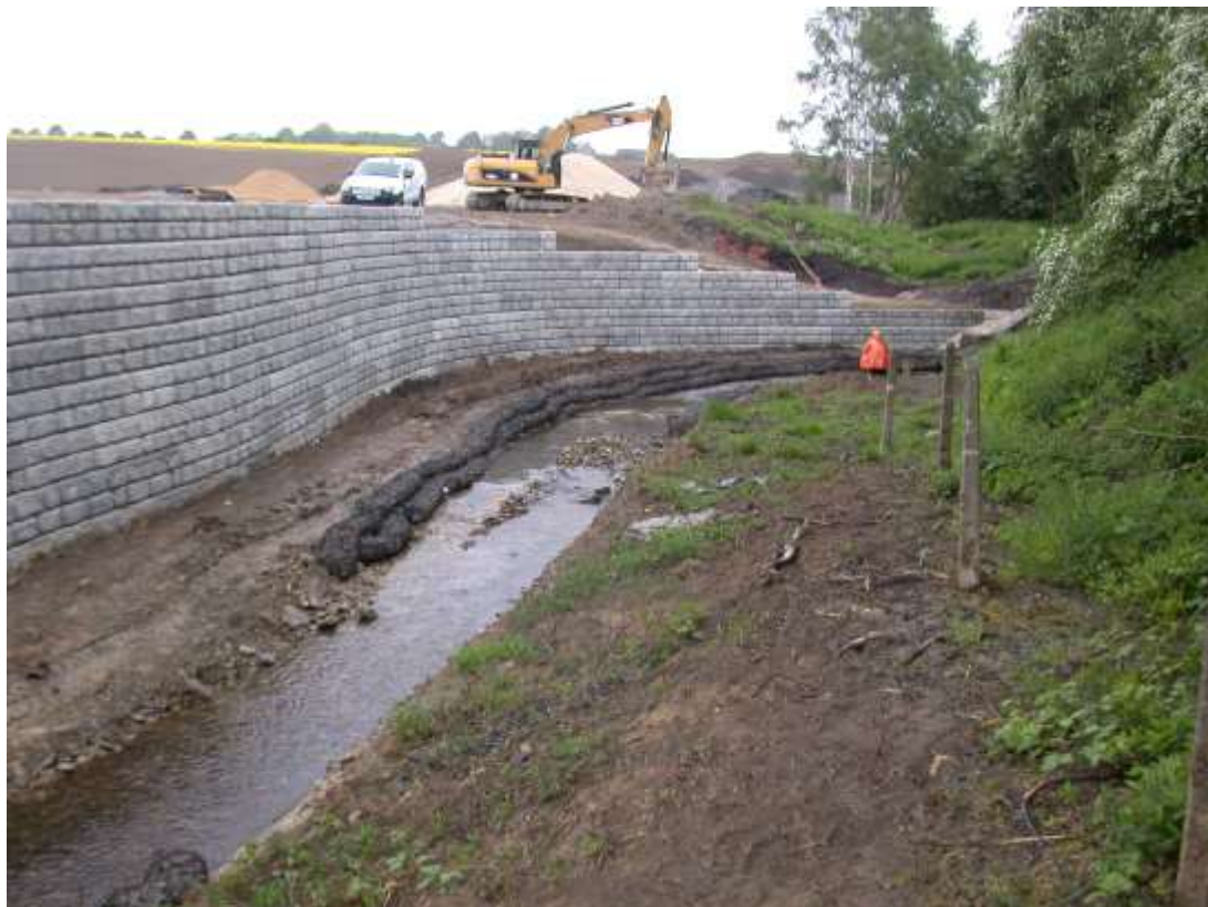
Diversion of the Hawke Brook and construction of a retaining wall to create development plot above.
