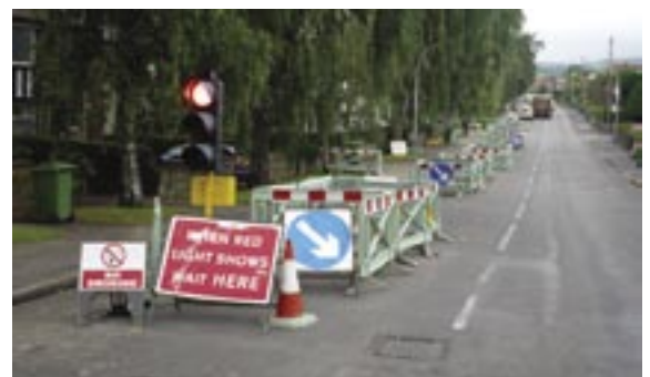
Utility highway excavations.
