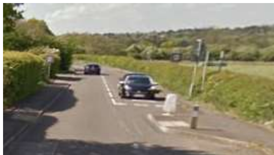
Image 10: Example of build-out environmentally damaging measure
