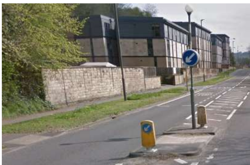
An island refuge which is obtrusive in the street scene but is positively acting as a pedestrian crossing point
