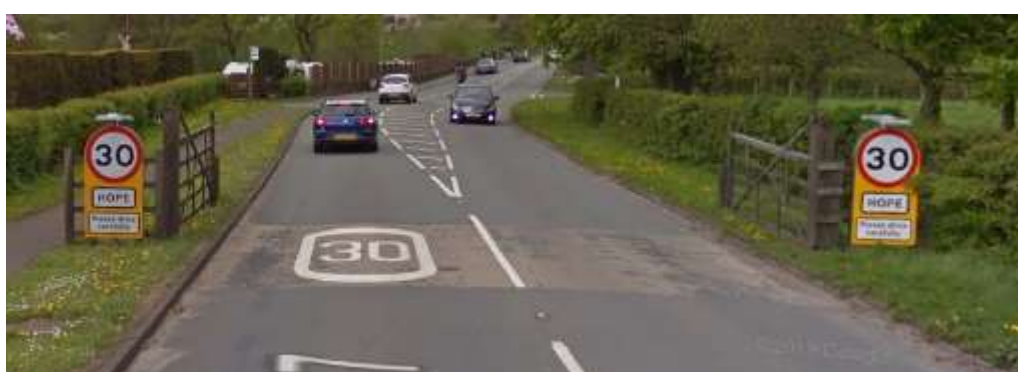
Image 5: Example of a gateway environmentally undesirable measure
