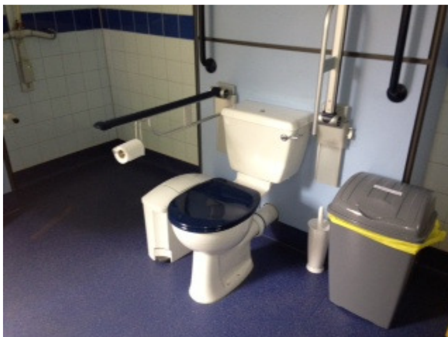
The toilet with access to both sides
