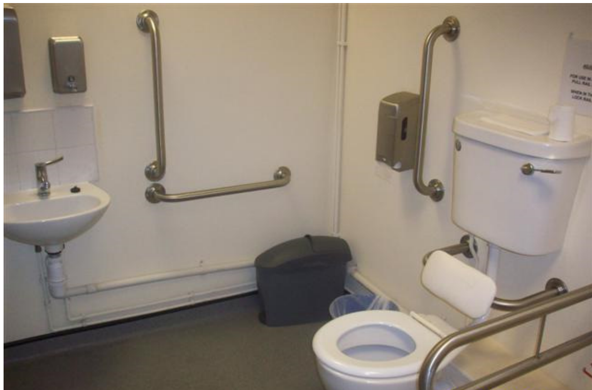
Toilet with space either side for assistance
