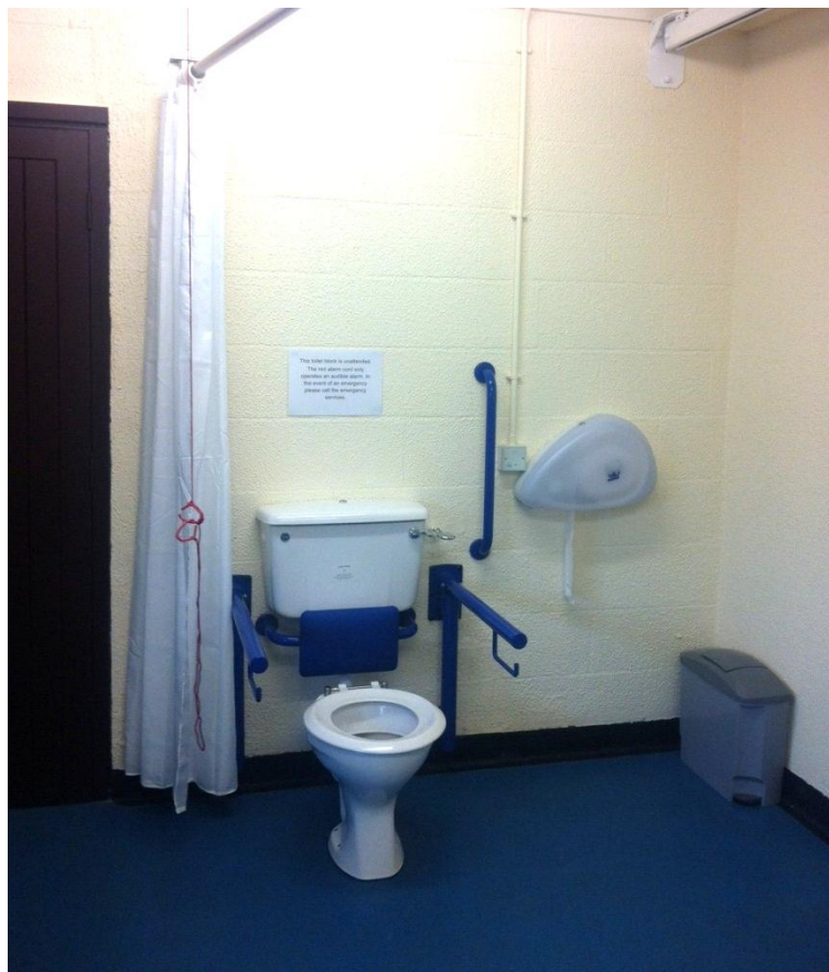
Toilet with space either side and privacy curtain
