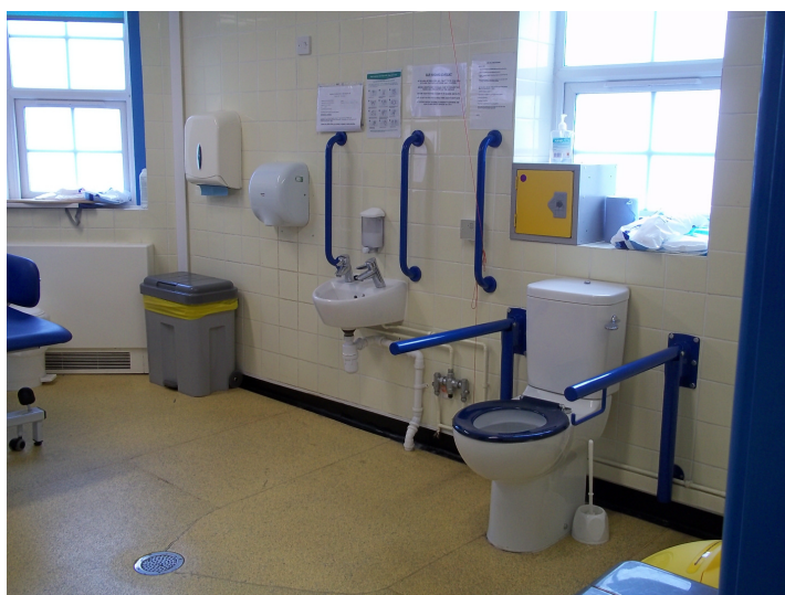
Toilet with space for assistance
