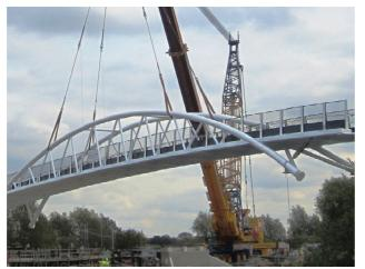
Putting into place the last piece of the **Trent Valley Greenway** jigsaw, with a new 12 tonne steel bridge over the River Erewash at Trent Meadows. This provides walkers, horse riders and cyclists with a safer, more direct link from Long Eaton
