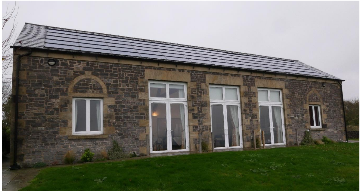
Over Haddon Village Hall, Derbyshire: Solar PV and air source heat pumps, within the Peak District National Park and on the edge of the Over Haddon Conservation Area. Image with permission of Over Haddon Village Hall.
