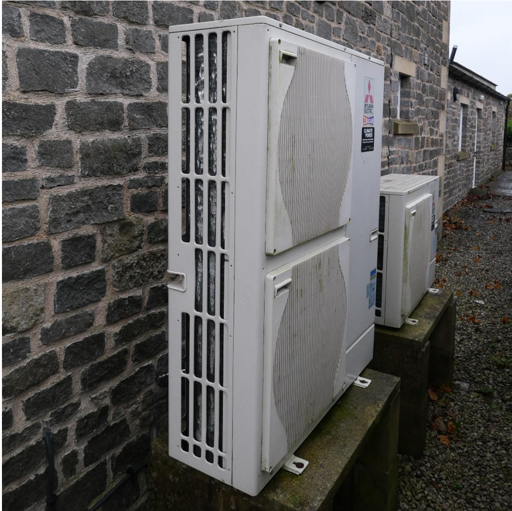
Air source heat pumps, Over Haddon Village Hall, Derbyshire. Image with permission of Over Haddon Village Hall.
