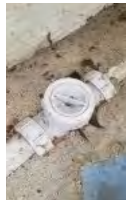
Puddle sucker, non return valves added to all the pipe work and sump pumps in the outhouse.
