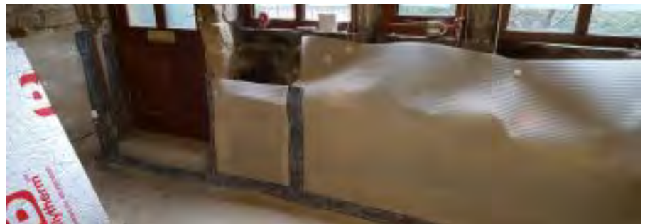
Waterproof membrane during installation.
