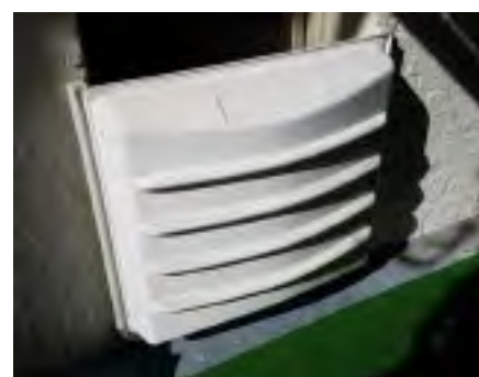
Flood barrier on the back door.
