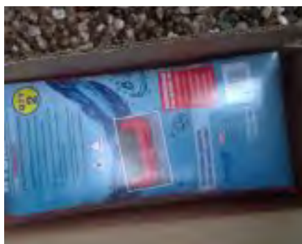
Absorbent packs swell up and block water.
