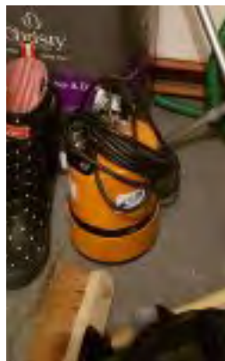
Puddle sucker, non return valves added to all the pipe work and sump pumps in the outhouse.
