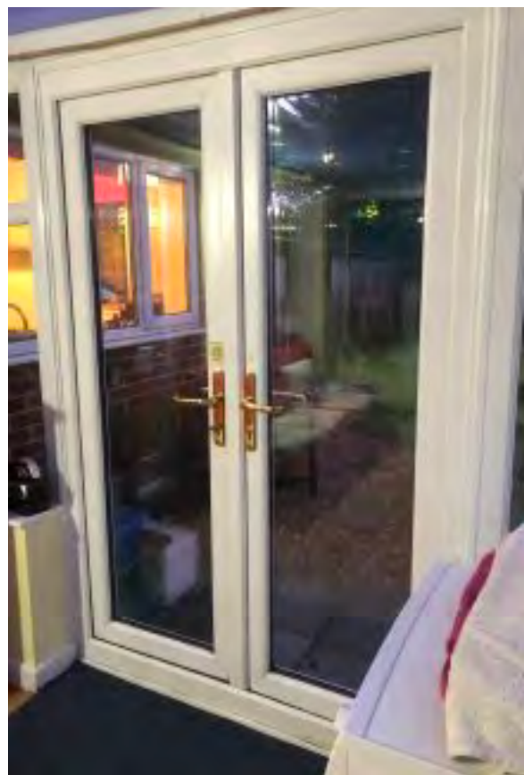
Flood resilient patio doors have been installed.
