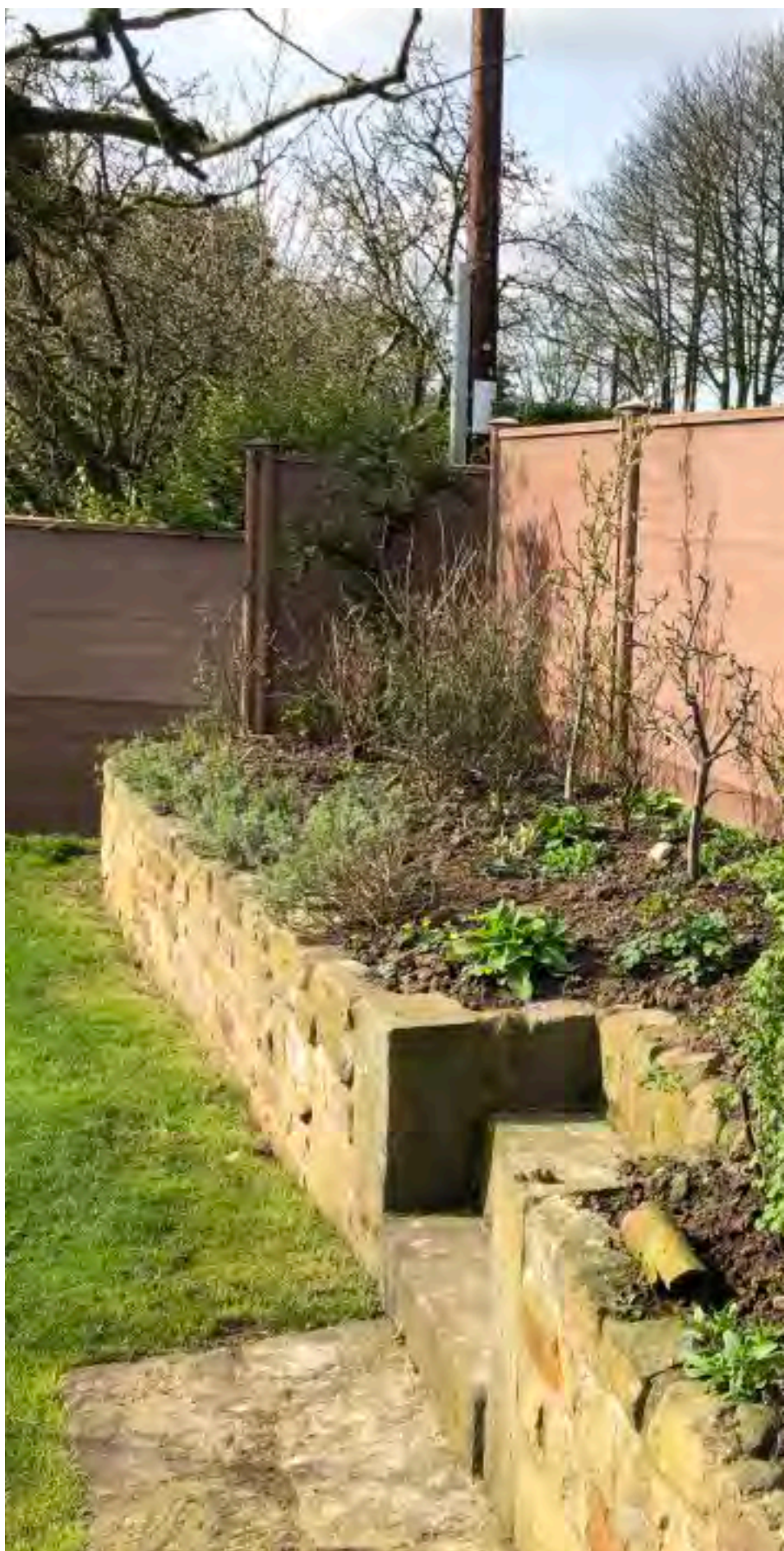
At the perimeter of the garden one-metre-deep holes were filled with concrete, into which posts and reinforced 'Task Green' waterproof fence panels were fitted.
