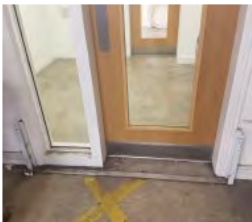
Flood barriers to all doors and UPVC door architraves.
