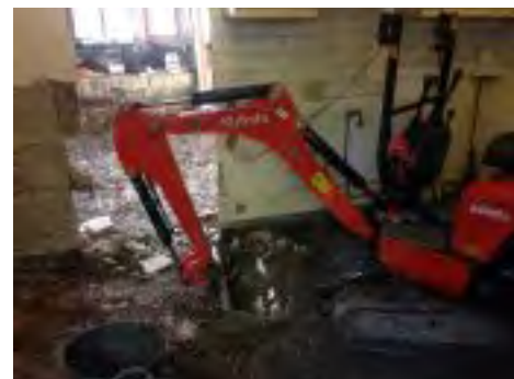
The rebuild involved excavating and 'tanking' the whole of the ground floor
