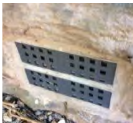
Self-closing airbricks.
