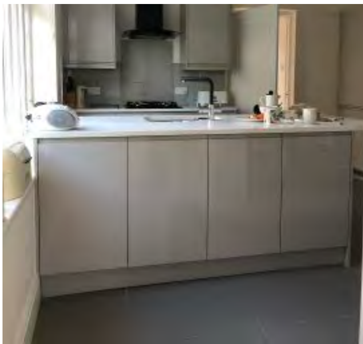
The kitchen is on legs with removable kick boards.
