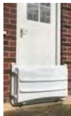
Electric sockets further up the walls, barriers to all external doors and non-return valves fitted.
