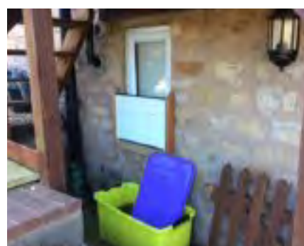
Flood barrier to basement door and window.
