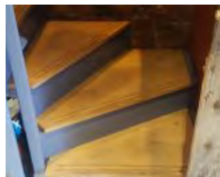
Steel staircase and solid oak treads.
