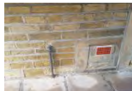
Walls were repointed and coated with a water proof spray and self-closing airbricks fitted.
