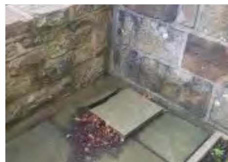
Sump created, into which powerful submersible pump can be dropped when flooding commences.
