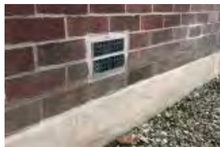
Self-closing air bricks and waterproof rendering was applied underground to the foundations and 30cm above ground.
