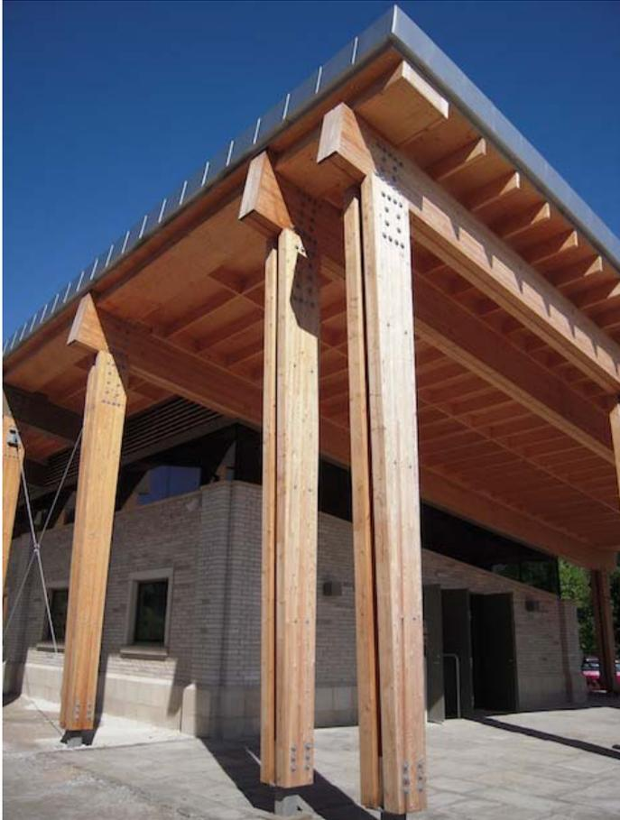
The timber frame is supporting the whole roof and is made from Siberian Larch, which grows very slowly in harsh conditions. This gives it a natural oil so no preservative is needed.
