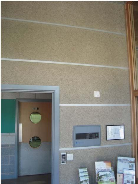
The remaining internal walls are constructed from an ecological board made from strands of wood bound together with minerals which are certified ecobiocompatible.
