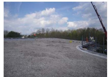
In total there is approximately 160tons of material on the roof so you can see why the roof timbers have to be strong.
