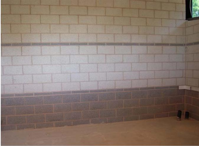
The internal walls are heavily insulated with recycled mineral wool and finished with an Enviromasonry building block that is manufactured in the UK from over 65% recycled aggregate under strict environmental and social legislation.
