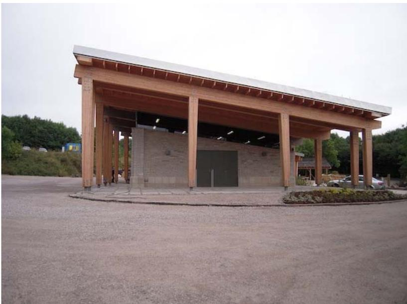
The external walls are non-load bearing and are constructed from natural Derbyshire stone. The coursed stone is cut limestone from Longcliffe, which demonstrates two techniques.
