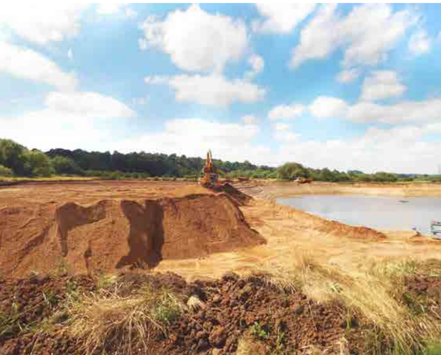
Shardlow Quarry - sand and gravel extraction
